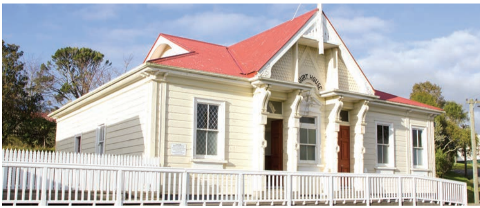
Right: The Stratford Court-house: 1990 and now.
